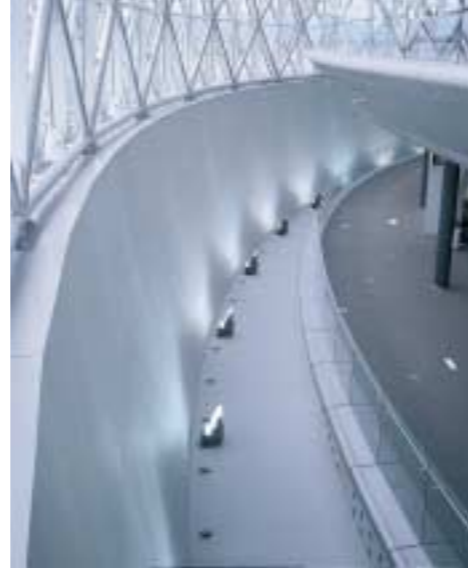
13 above: Inside the dome perimeter, showing the space between the dome and the internal floors.
