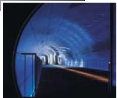
7. Looking into the submerged tunnel from the entrance building.
