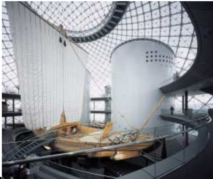
16. The higaki kaisen surrounded by the annular floors. The ship sits on reinforced concrete columns with seismic isolators.
