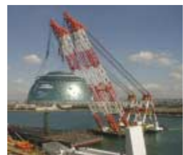
(b) Lowering the dome onto the barge.
