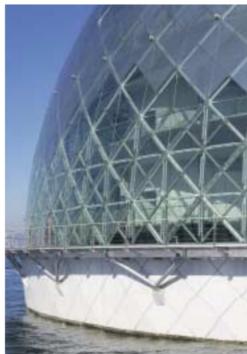
5. The escape deck at the dome's 'equator': behind the glass are the structural T-sections, designed for resistance to wave impact.
