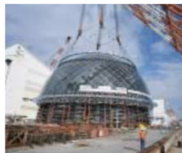
(a) Lifting the 1200 tonne dome from the propping jigs.
