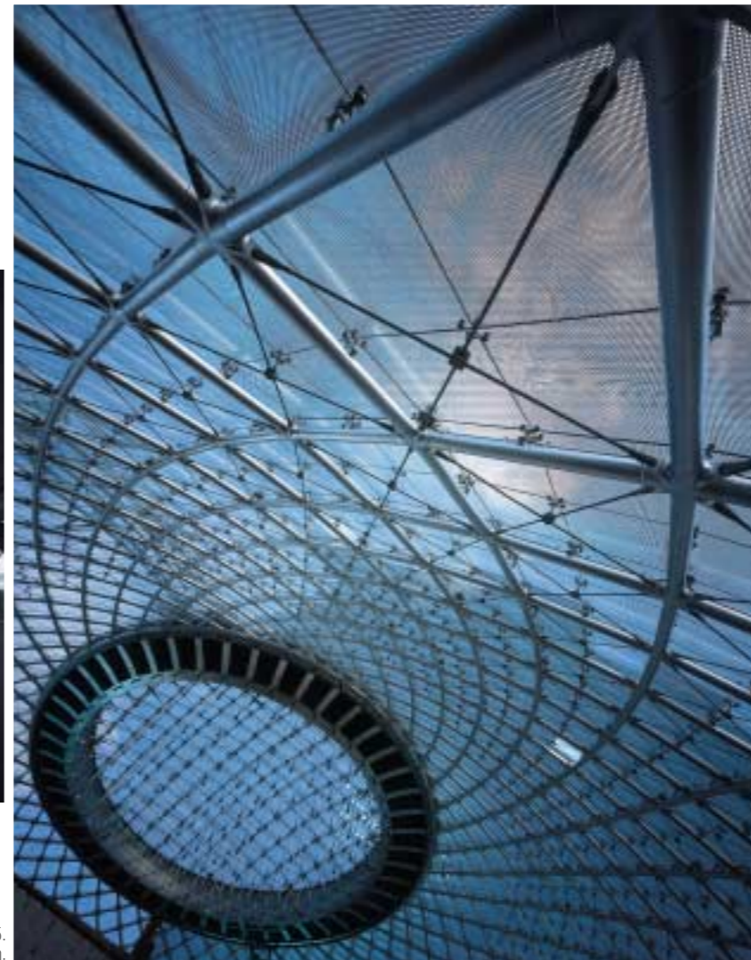
15. The diagrid shell and the ring beam.
